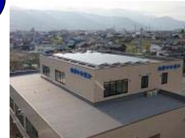
Solar power unit
