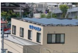
Solar power unit
