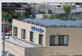
Solar power unit
