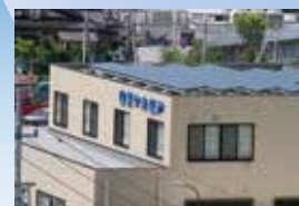
Solar power unit
